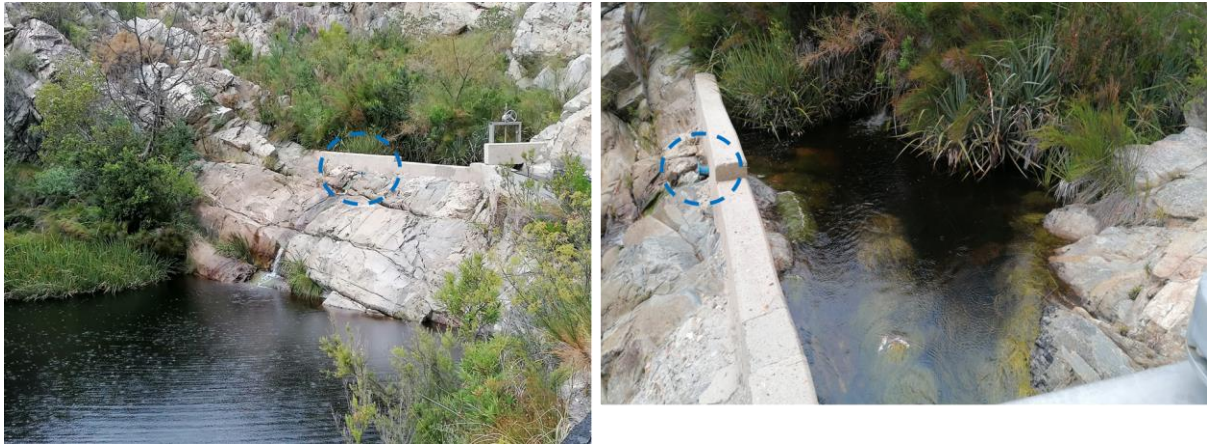
Figure 8: Pictures showing the small pipe (release valve) that was installed at the water take-off point in the upper Huis River as a measure to prevent complete abstraction and maintain stream flow below the water take off point. Pictures: Aileen Anderson (Grootvadersbosch Conservancy Trust (GVBCT)).
